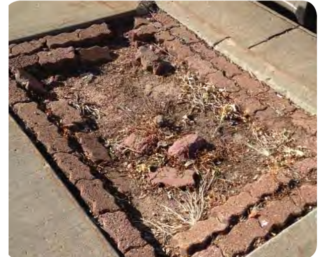
Deteriorated Pavers
