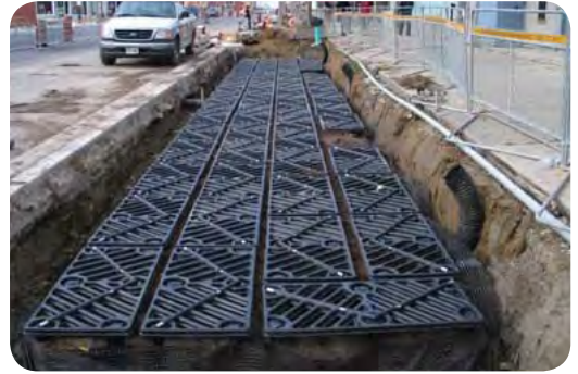
Silva Cell System being installed
