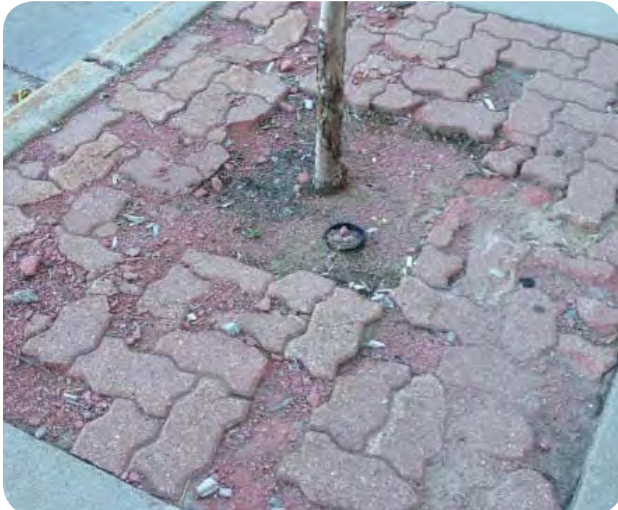
Deteriorated Pavers
